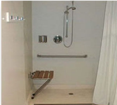
Shower controls adjacent to fixed bench
